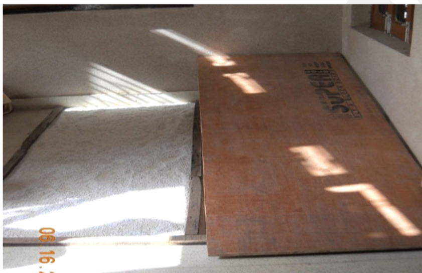
Figure 3(e): Marble chips and ramp
